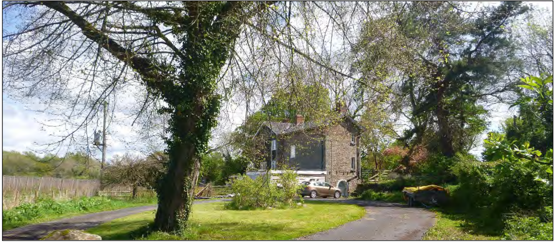
Photograph 12 View south of Lock Cottage from the top of the driveway
