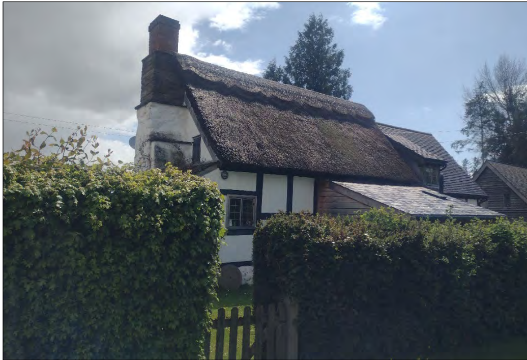
Photograph 10 View south of Thatch Cottage from the road
