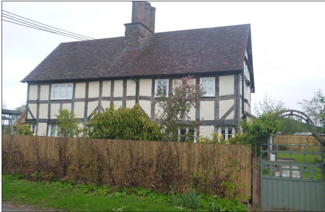
Photograph 7 Southern aspect of Old Dairy, from the road
