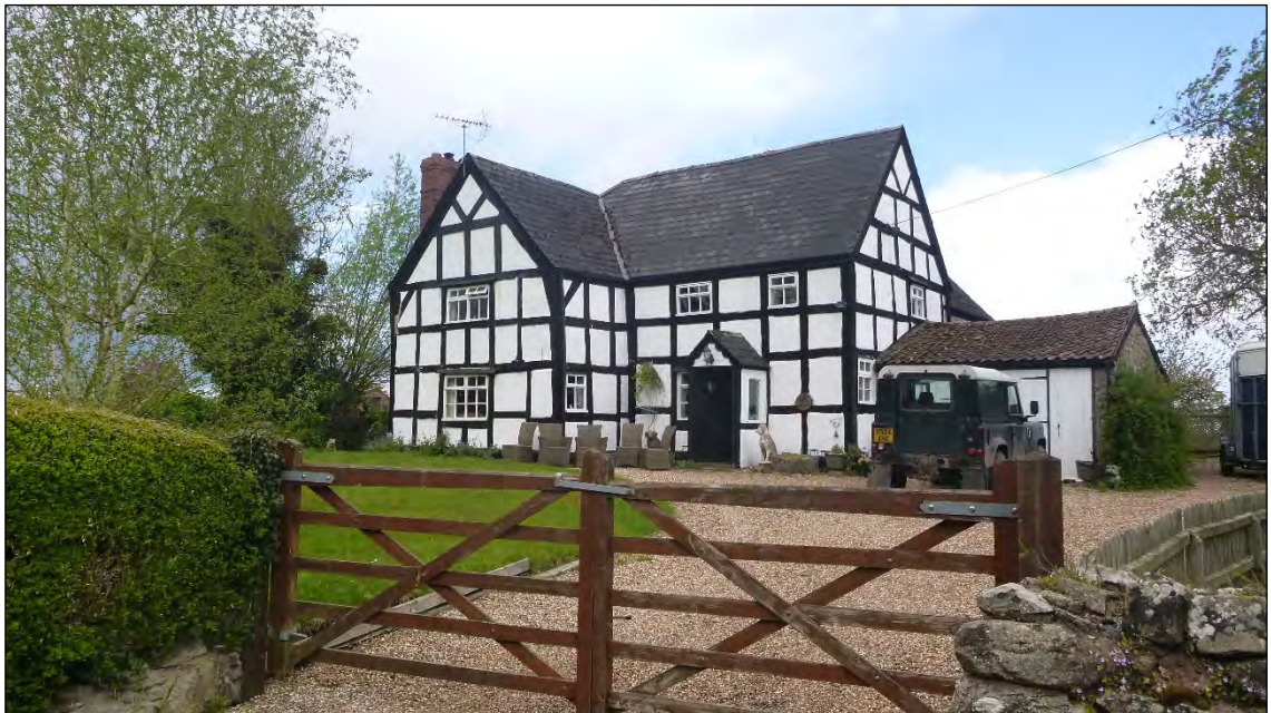
Photograph 5 The Post Office from the road, looking west
